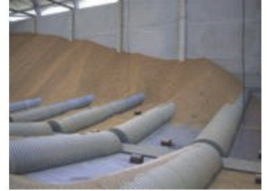
1m wide semicircular aerating ducts. Potential reclaim capacity on paddy rice: 500t/h.
