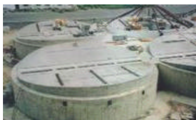
Concrete base sloped for the Vibrafloor elements
